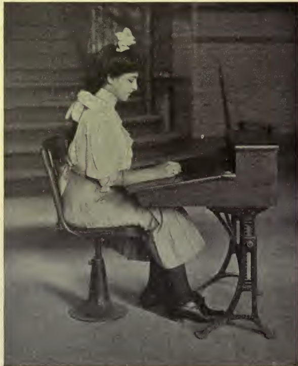
FIG. 38.—ADJUSTABLE DESK WITH NARROW BOX; BOTH SEAT AND DESK ARE ADJUSTED TO THE PUPIL WHEN SEATED.
